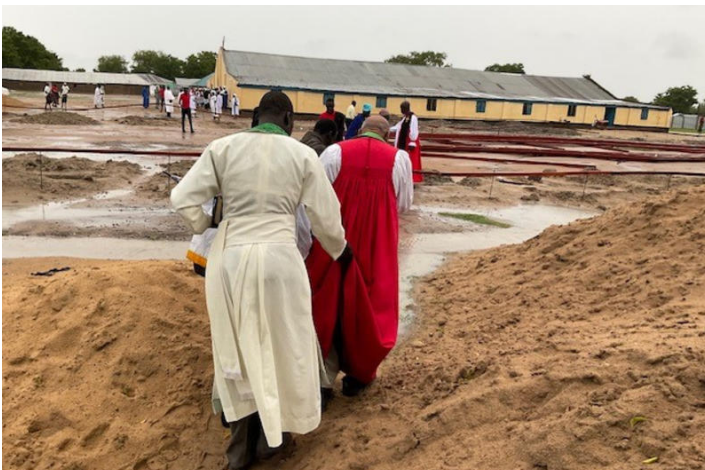
Navigating building work in progress for a new cathedral
